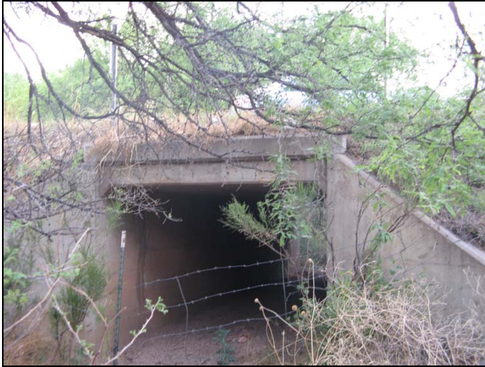
Figure 10: A 10x10' box culvert blocked by barbed wire at Waypoint 30, Milepost 18 on SR-82
