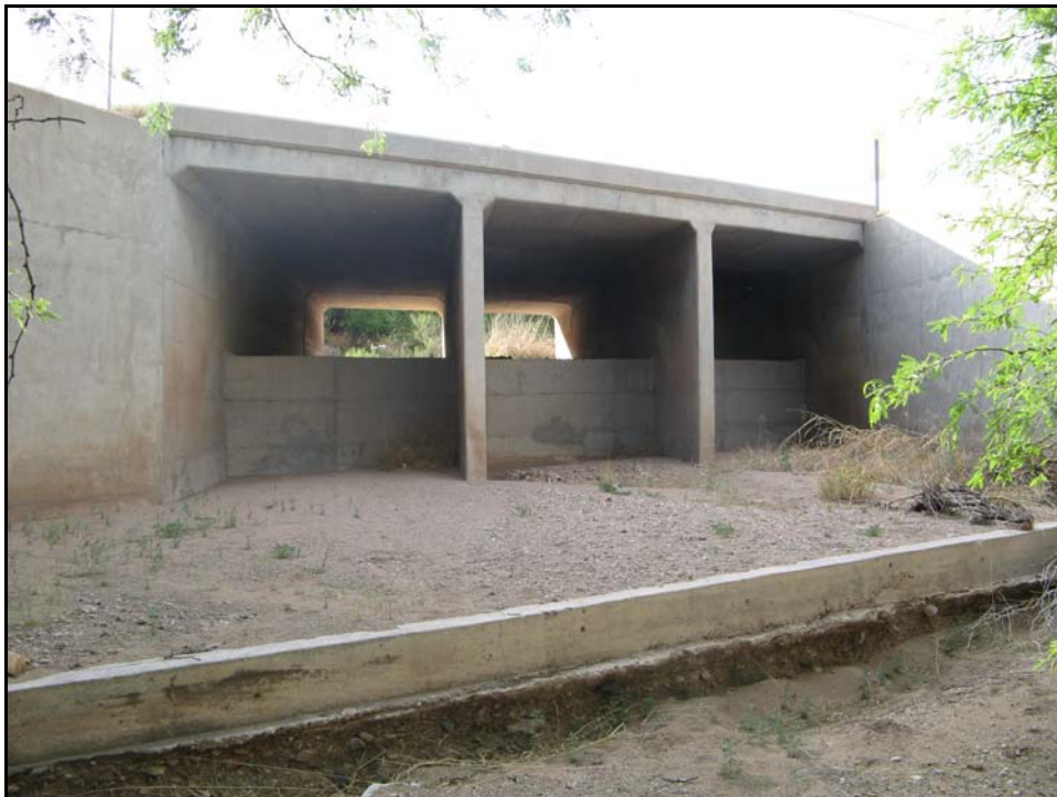
Figure 11: 5x6' pour-offs in 3 box culverts at Waypoint 33, Milepost 21.7 on SR-82
